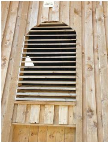
Vertical and horizontal treated sawn timber boarding to warehouse and barn
